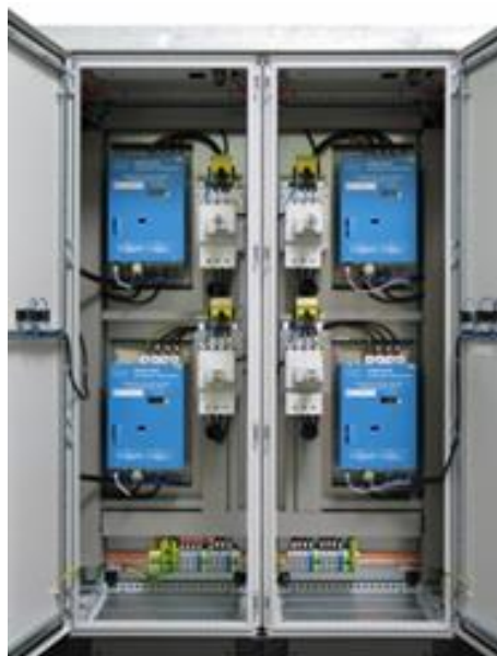
Fig. 10-11 Control cabinet with four medium-frequency inverters with individual main switches
